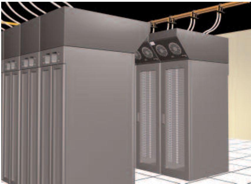
An open approach to supplemental cooling supports can support higher equipment densities across the facility.
